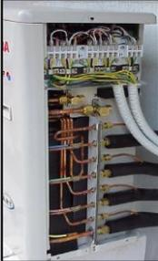
The photograph shows the internal components of an inverter air conditioning unit, including a rotary compressor and various electrical connections.
