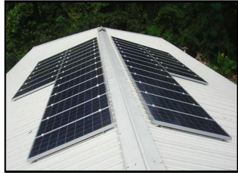
The roof area shaded by the panels amounts to just over 40 square metres, and is 10% of the total roof area.
