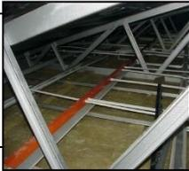
The photograph shows the underside of a ceiling, revealing a dense, fibrous rockwool insulation blanket installed between the ceiling joists.
